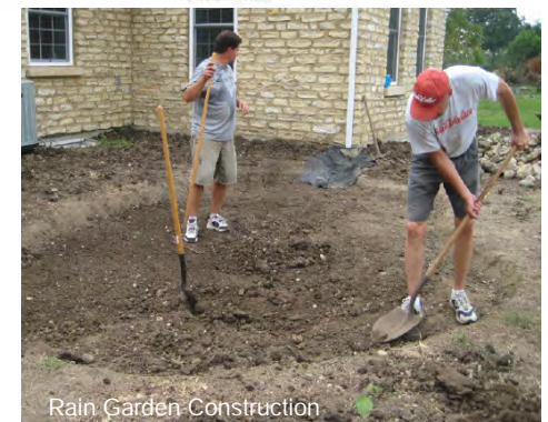
Rain Garden Construction
